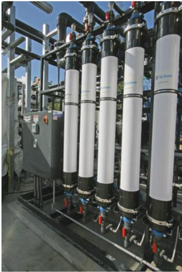
Ultrafiltration is key to the advanced purification process. Recycled water passes through ultrafiltration membrane modules (Scinor).
