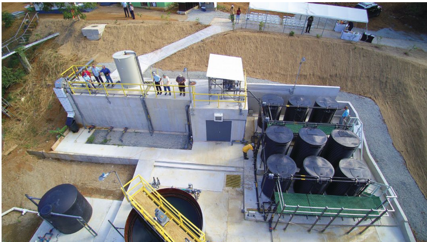
Fluence Corporation developed the membrane aerated biofilm reactor beginning in 2008. Its first US installation as a wastewater treatment plant is in Bordeaux, St. Thomas, US Virgin Islands.
