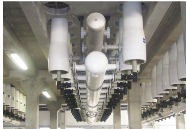
Lower portion of Sorek’s vertical RO pressure vessels
